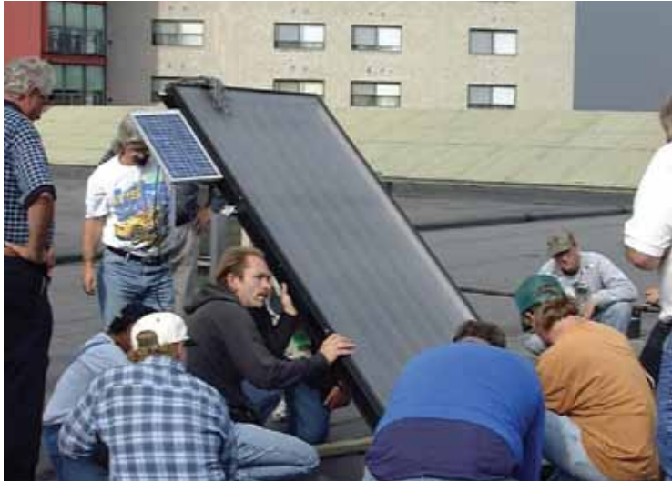
▲ Crew installing a solar panel for a solar hot water system
