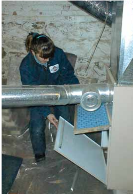
▲ Weatherization technician installs new furnace filter in a home in Vermont
