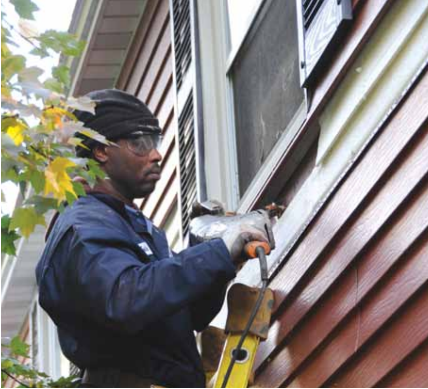
▲ Weatherization technician drilling siding for sidewall insulation
