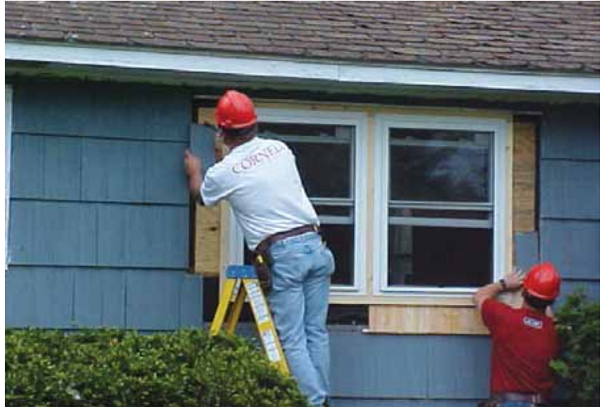
▲ Weatherization technicians repair and seal around windows
