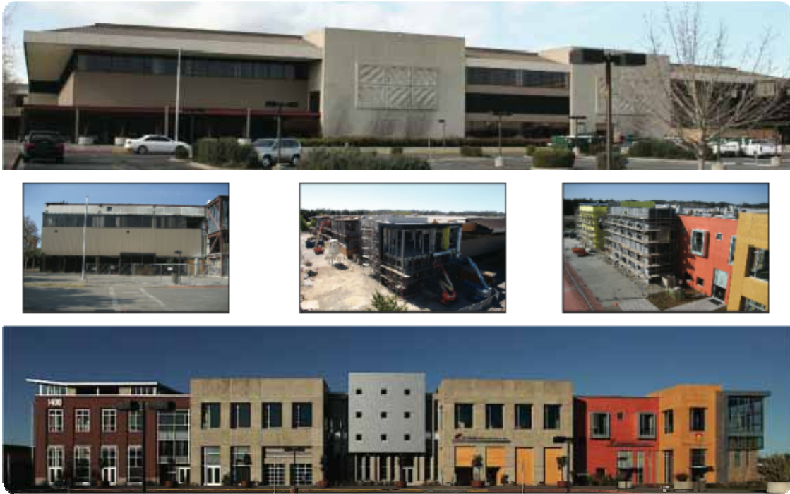
Timelapse photos of the adaptive reuse of an existing commercial building at Sonoma Mountain Village, using Coddling Steel Frame technology.
